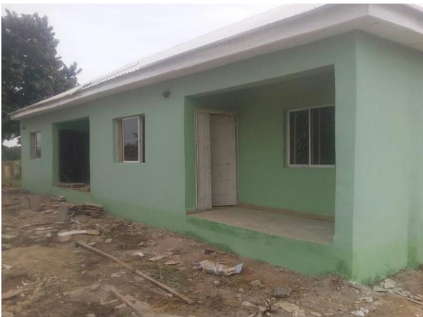
Renovated Staff quarters at Health facility in Gombi LGA, Adamawa. Photo:NRCS
