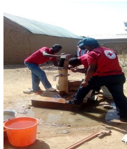
NRCS volunteers rehabilitating waterpoint in Kwarwa community at Gombi LG. Photo NRCS.
